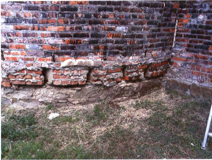
PICTURE 7 Back of Rotunda showing slots in brick for floor beams.
