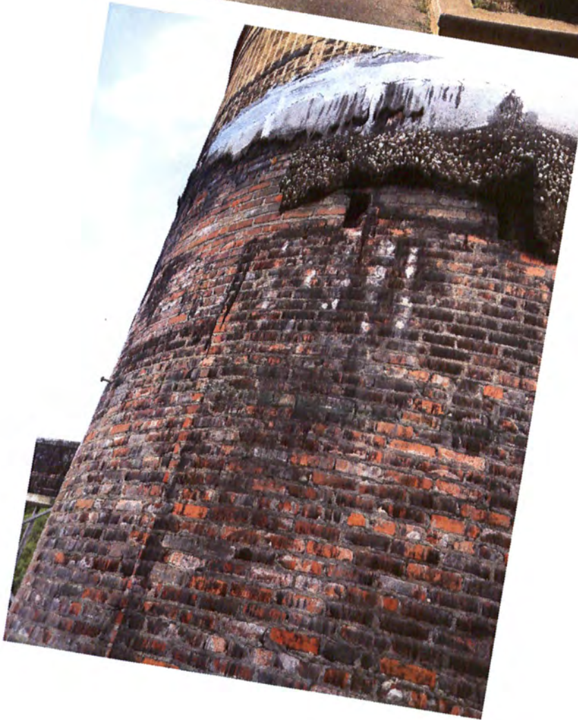
PICTURE 6 Back of Rotunda showing slots in brick for roof beams.
